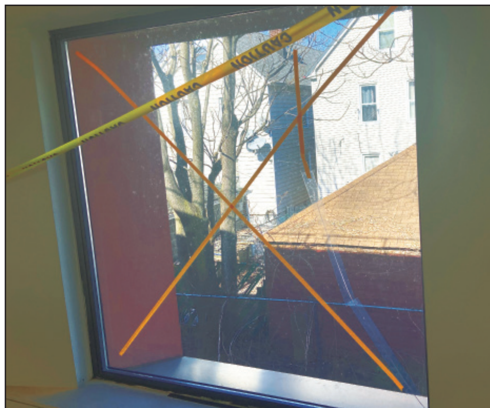
A cracked window in the Visual Arts Building on the second floor.
